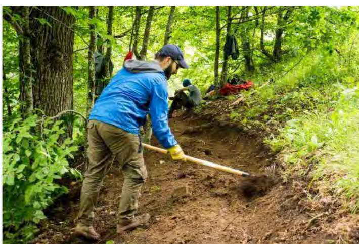
Rehabilitation and construction of the trail (Source: https://transcaucasiantrail.org/ )
