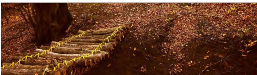
Construction of brifges by TFC (source: https://www.trailsforchangengo.org/ )
